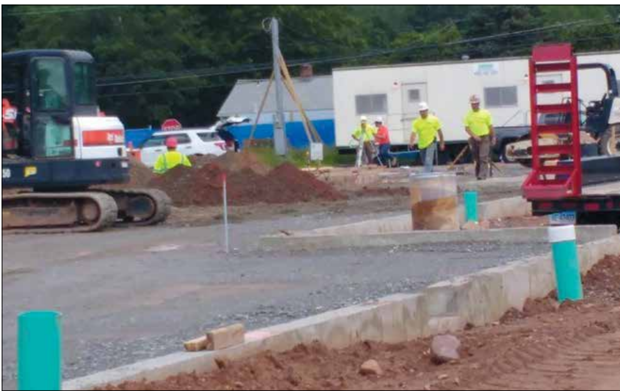
Construction is right on schedule!
